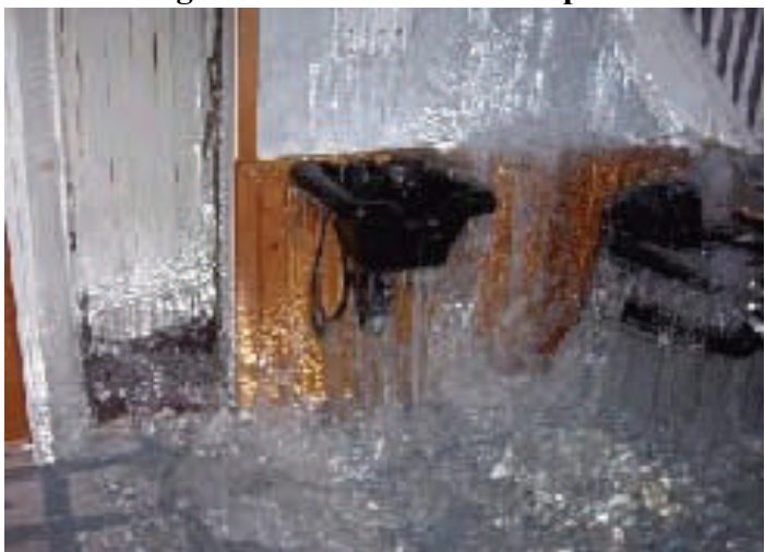
Damage can be excessive and expensive
